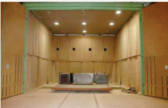
Enclosed grit blasting room
